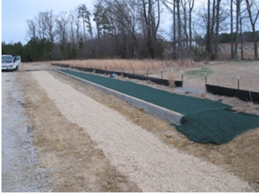
Figure 3.53 Level Spreader (CFB Contracting LLC 2019).
