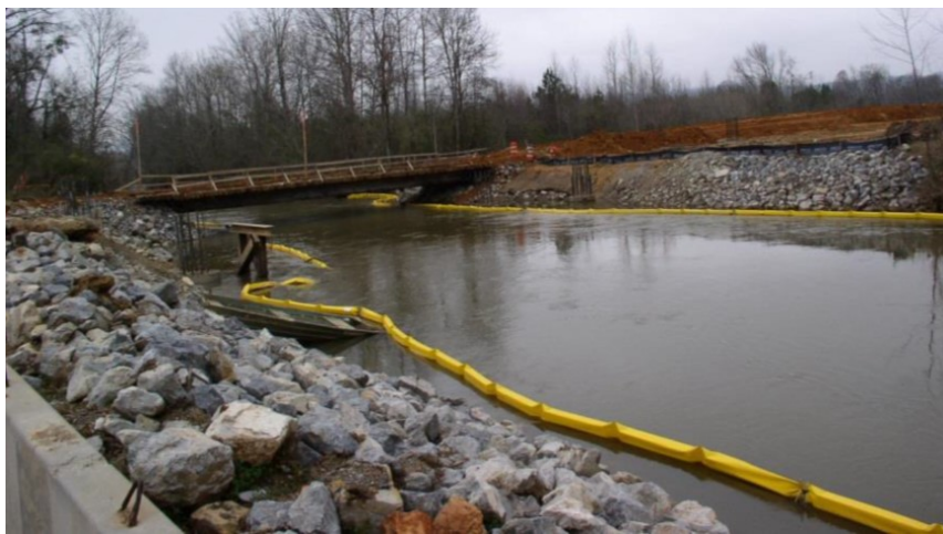
Figure 3.70 Turbidity Curtain (Alabama SWCC 2009).
