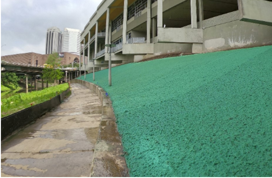
Figure 3.12 FGM on Slope after Application (Construction ECO Services 2019)
