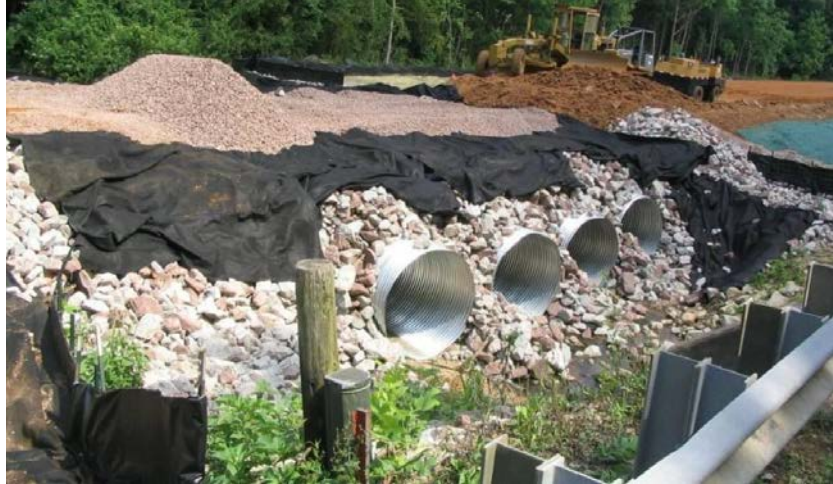
Figure 3.34 Temporary Culvert Crossing at Development Stage (TDOT DM 2012b).
