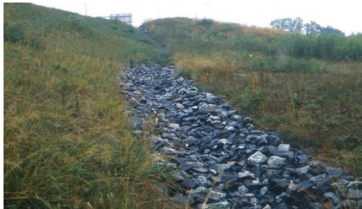
Figure 3.41 Rip-rap Lined Swale (OH DNR 2016)
