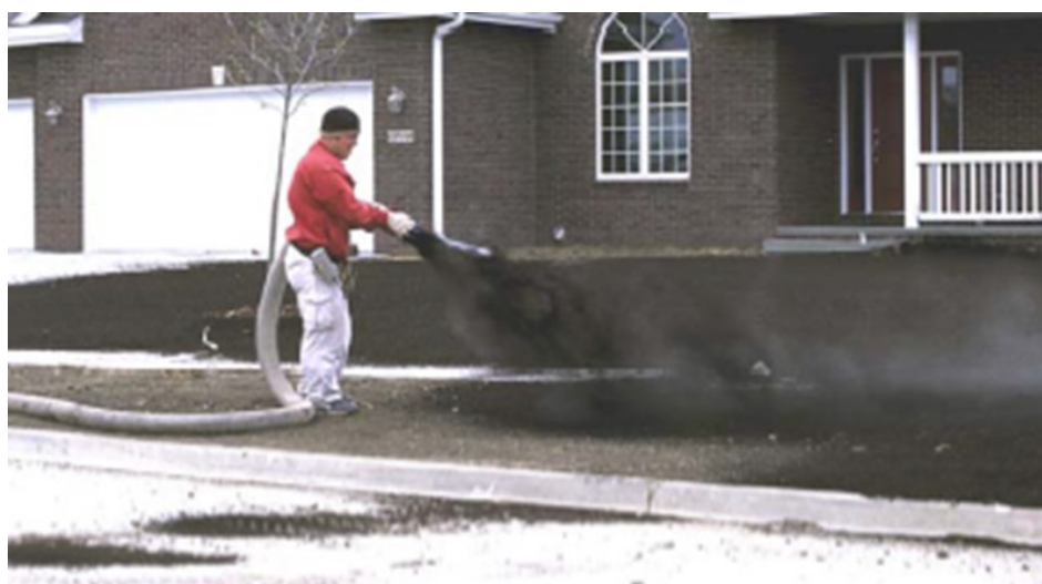
Figure 3.10 Compost Mulching Process (Indiana DEM 2007)
