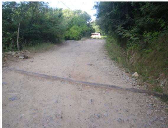
Figure 3.37 Water Bar Installed on Road (St. John Tradewinds 2019).
