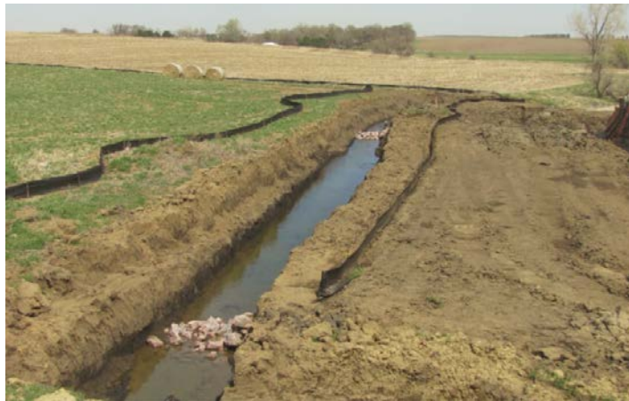
Figure 3.31 Temporary Stream Diversion. (Iowa DOT 2017).
