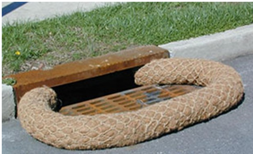
Figure 3.55 Storm Drain Inlet Protection (Eastcoast Site Work Inc 2019).
