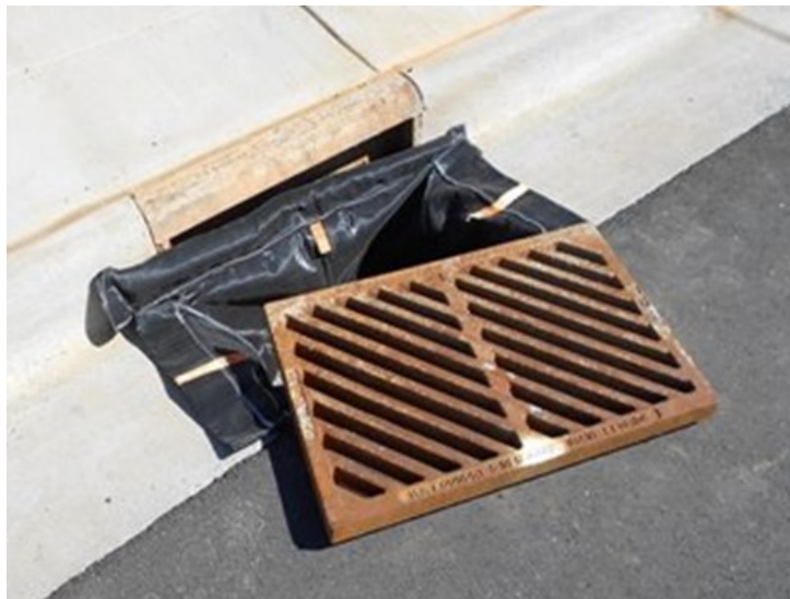
Figure 3.62 Inlet Filter Bag (Hanes Geo Components 2019).
