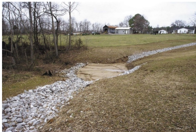
Figure 3.45 Rock Lined Channel (Kentucky DOC&DOW 2005).
