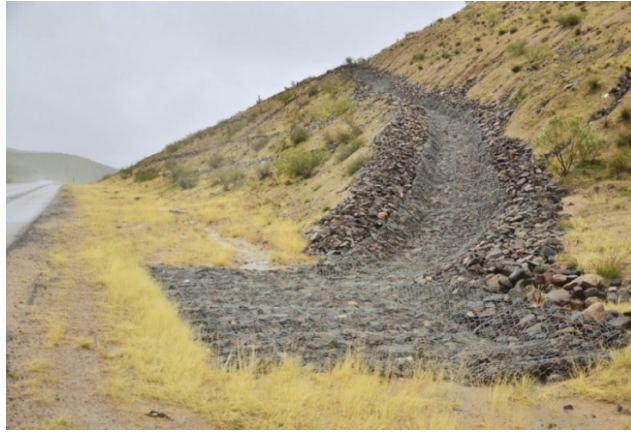
Figure 3.38 Gabion-style crown ditch (Arizona DOT 2012).
