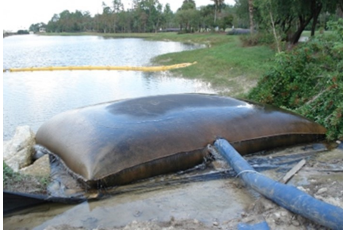
Figure 3.79 Pumped Water Filter Bag. (Midwest Construction Products 2019).
