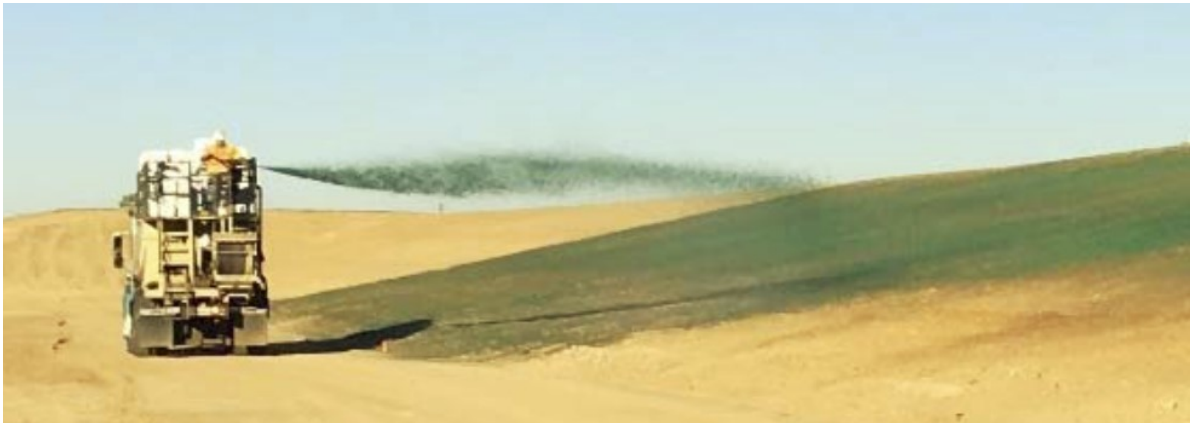
Figure 3.29 Hydroseeding Application on a Slope (Caltrans 2017)
