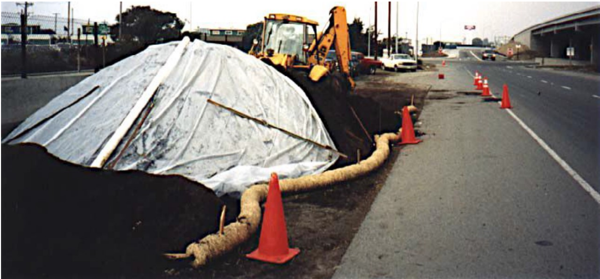
Figure 3.7 Stockpile Management at a Construction Site (RI SCC 2014).
