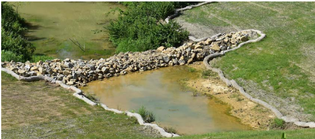
Figure 3.49 Rock Check Dam with perimeter barriers around the upstream basin.
