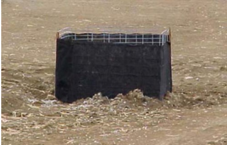
Figure 3.59 Geotextile Fabric Drop Inlet Protection (Indiana DEM 2007).
