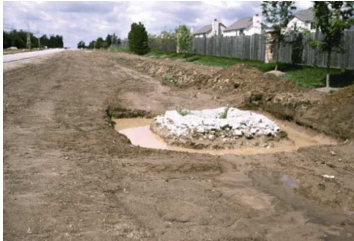
Figure 3.56 Excavated Drop Inlet Protection (Indiana DEM 2007).
