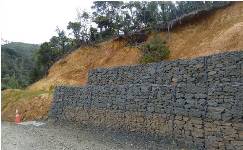
Figure 3.23 Gabions Installed to Protect Slope Failures (Cirtex Civil 2018).
