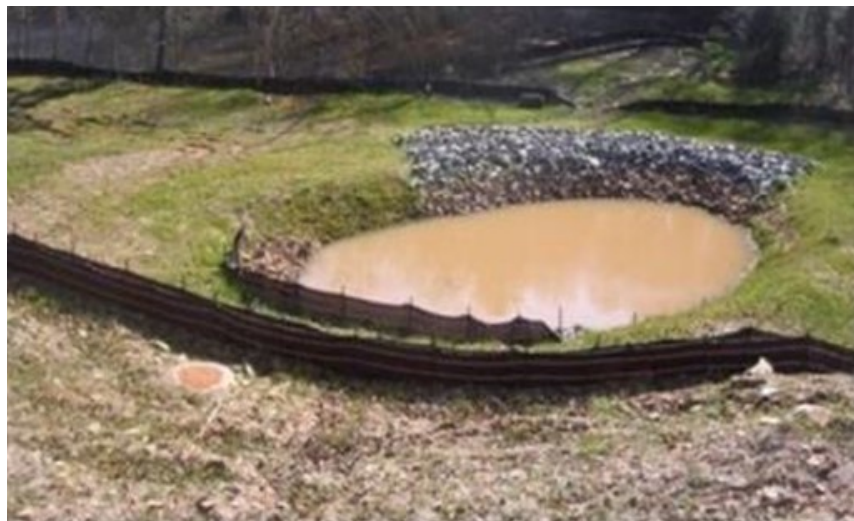
Figure 3.73 Sediment Trap (MN PCA 2019c).
