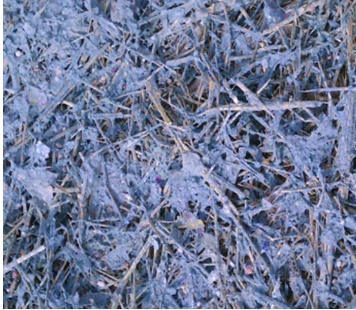
Figure 3.13 Bonded Fiber Matrix after Application (Ecosorb International 2019).
