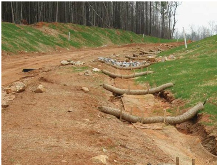
Figure 3.47 Staked Erosion Log Check dams (Scott and Rich 2015).
