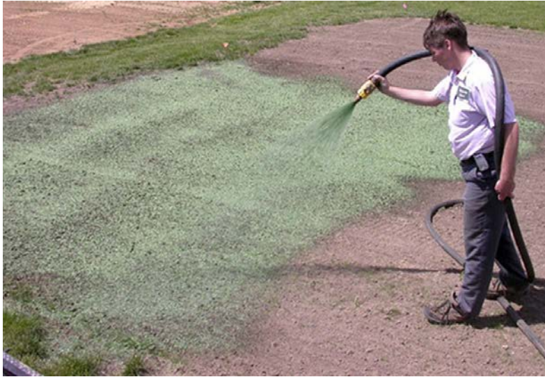
Figure 3.17 Application of Soil Binder along with Mulch (USDA 2014).
