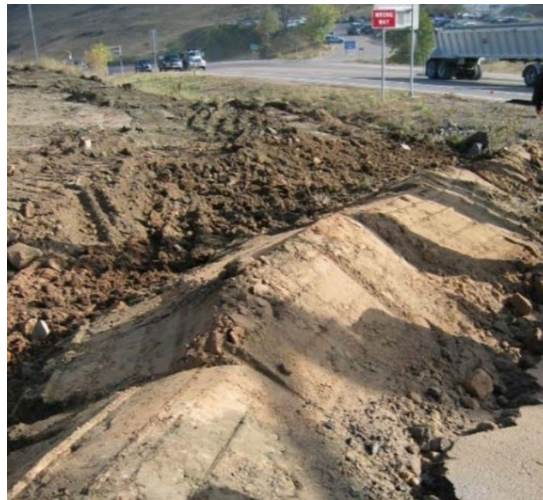
Figure 3.42 Temporary Berm Constructed with Compacted Soil (MN PCA 2019a)
