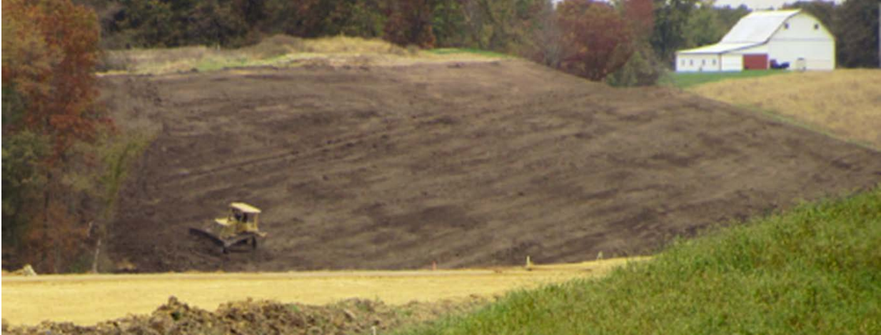
Figure 3.6 Topsoiling Practice (Iowa DOT 2017)
