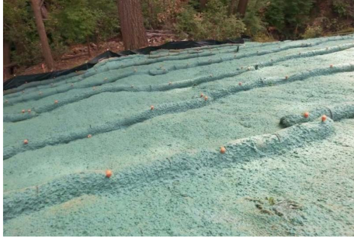
Figure 3.11 Slope after Application of Hydraulic Mulch (Caltrans 2017)
