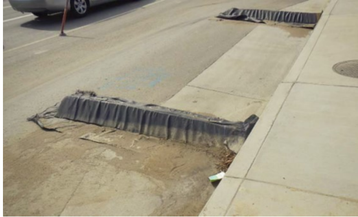
Figure 3.69 Flexible Sediment Barrier (Caltrans 2017).
