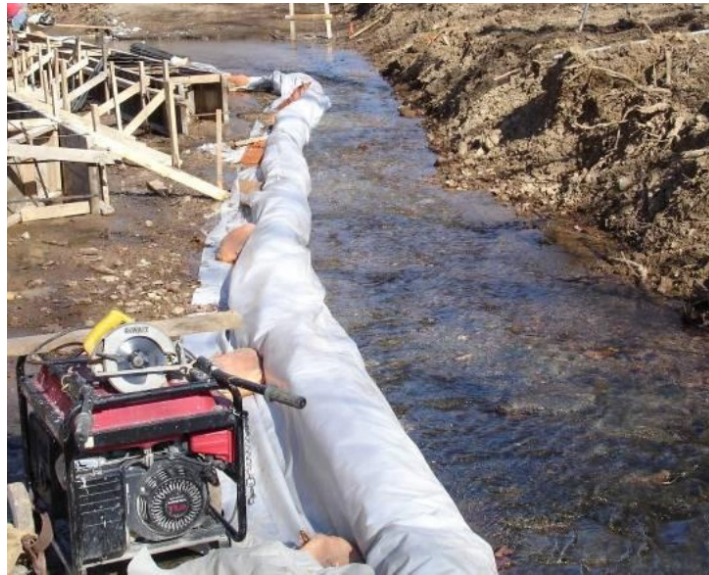
Figure 3.33 Temporary Instream Diversion at a Channel (TDOT DM 2012b).
