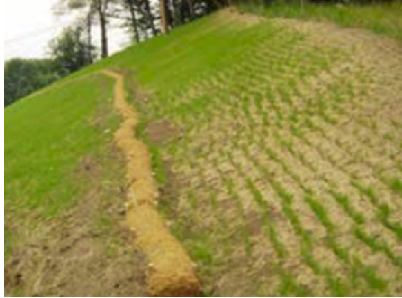
Figure 3.27 Fiber Rolls on a Slope (New York DEC 2016).
