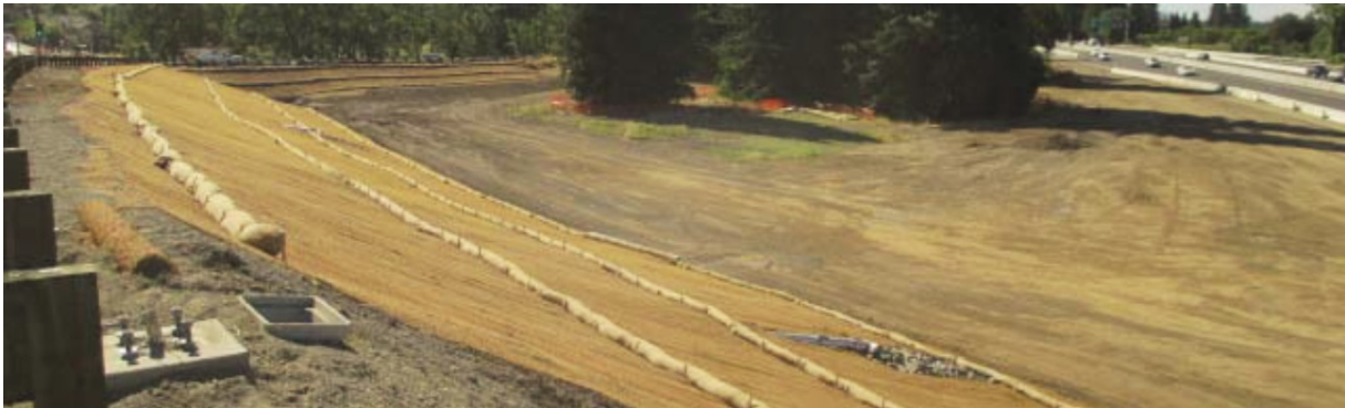
Figure 3.14 Slope after Application of Erosion Control Blankets (Caltrans 2017).
