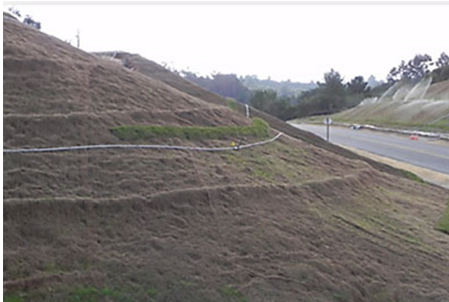
Figure 3.16 Compost on Slopes Covered by RECPs (Caltrans 2019a).
