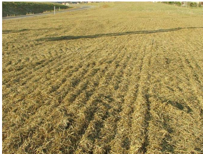
Figure 3.8 Land after Dry Mulch Application (WY DOT 2011).
