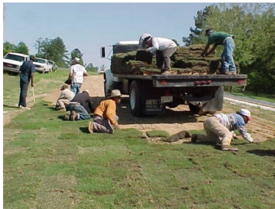
Figure 3.30 Sodding Application Process (Alabama SWCC 2009).
