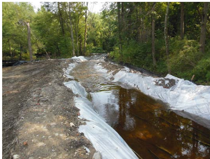
Figure 3.46 Temporary Lined Channel (Rachel Calabro 2012).
