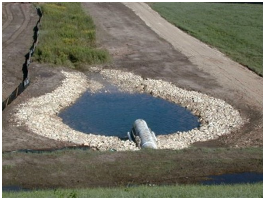
Figure 3.54 Plunge Pool (Minnesota Pollution Control Agency 2016b).
