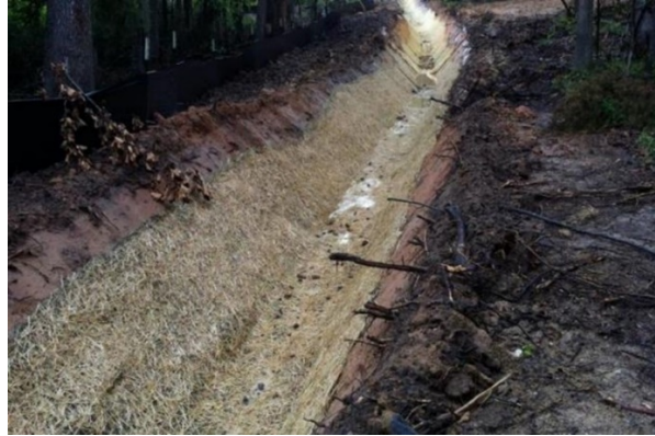
Figure 3.36 Permanent Diversion Ditch (Campco Engineering INC 2019).
