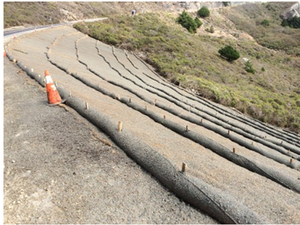
Figure 3.68 Wattles on Slopes (Superior Hydroseeding Inc 2019).
