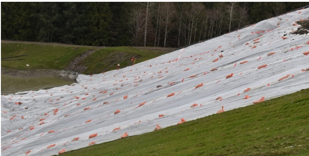
Figure 3.22 Temporary Plastic Sheeting on a Slope (Encore Environmental LLC 2019).
