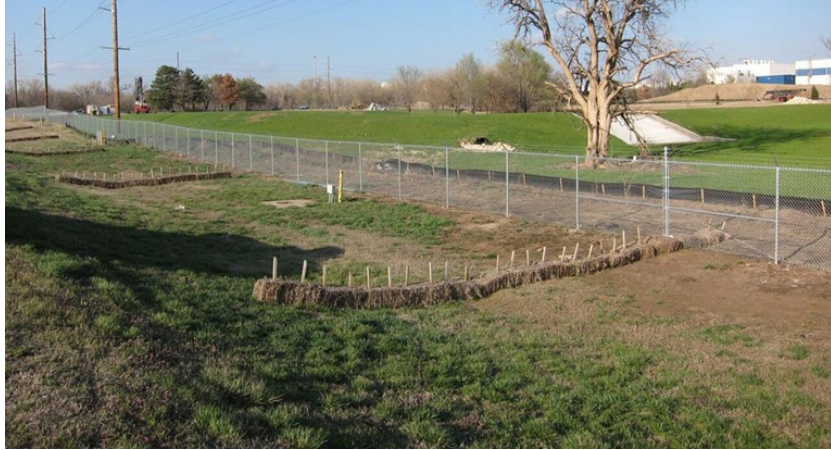
Figure 3.48 Hay Bale Check Dam (Challenger Construction Corp. 2015).
