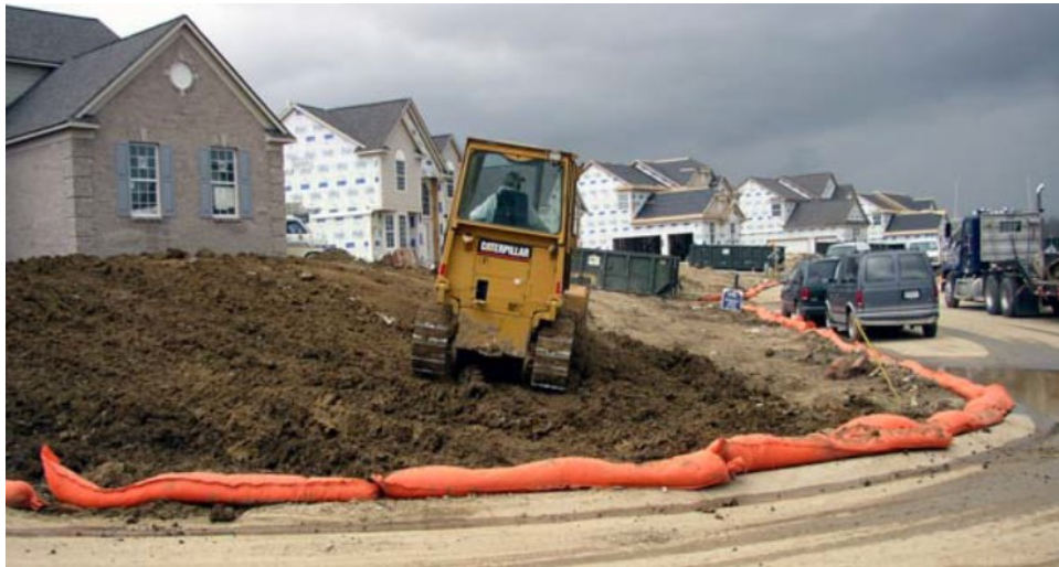
Figure 3.78 Perimeter Filter Barrier (Indiana DEM 2007).
