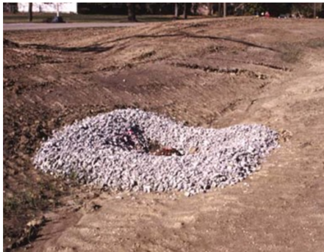
Figure 3.58 Gravel Donut Drop Inlet Protection (Indiana DEM 2007).
