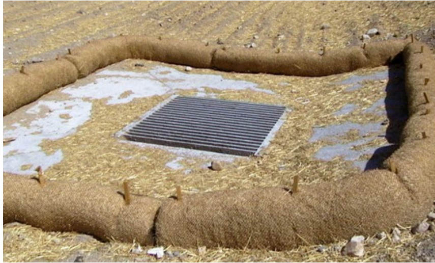
Figure 3.63 Wattles Used for Inlet Protection (Forestry Suppliers Inc. 2019).
