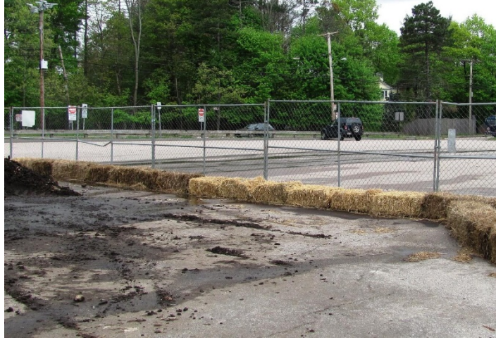
Figure 3.66 Straw or Hay bale Perimeter Barriers (Mass DEP 2019)
