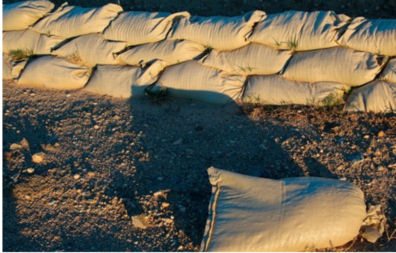
Figure 3.72 Sandbag Barriers (CCI SUPPLIES 2019).
