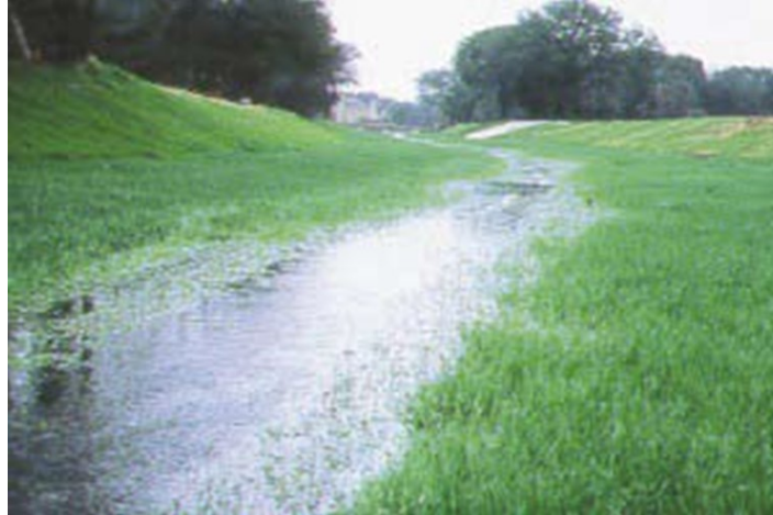
Figure 3.44 Grass-Lined Channel (Kentucky DOC&DOW 2005).
