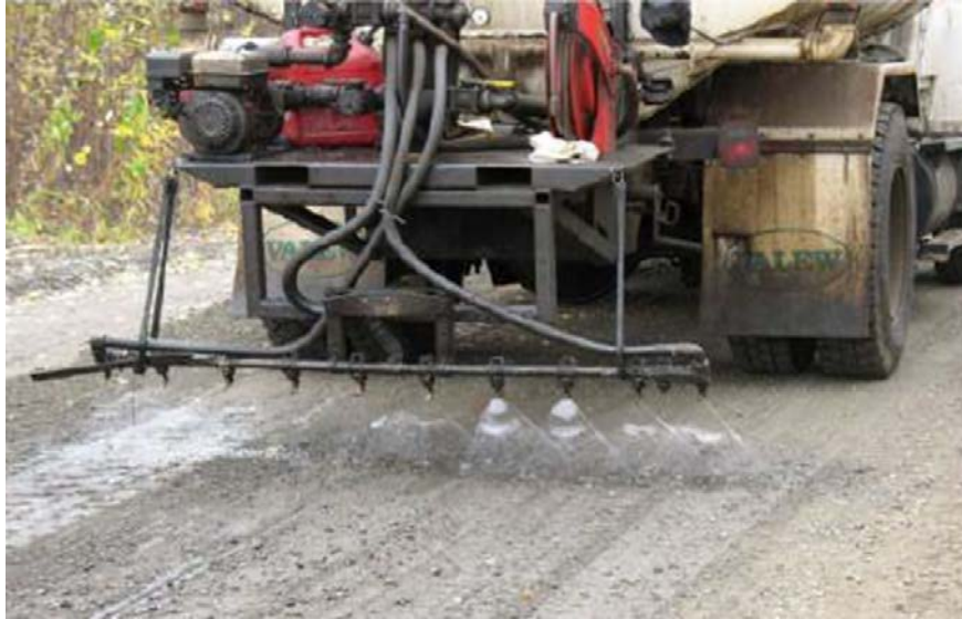
Figure 3.18 Dust Palliatives Application on a Gravel Road (Alaska DAQ 2012).
