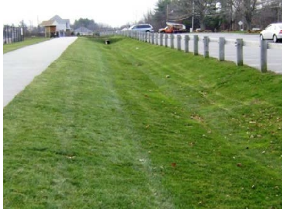
Figure 3.40 Vegetated Swale (Mass DEP 2019).
