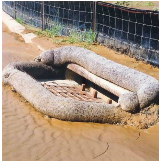
Figure 3.65 Curb Inlet Protection with Fiber Logs (1st Resource Solutions LLC 2019).
