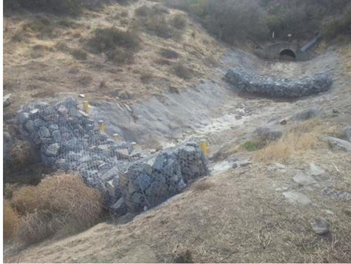
Figure 3.50 Gabion Check Dams (Gabion Supply 2019).
