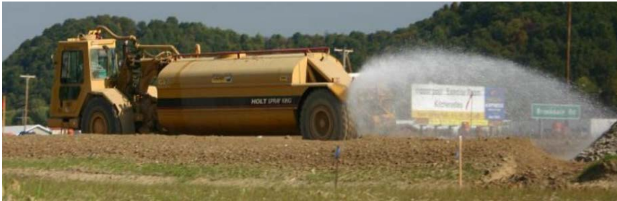
Figure 3.5 Watering at a Construction Site to Control Dust (TDOT DM 2012b)
