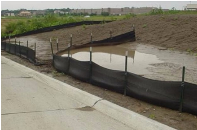
Figure 3.71 Perimeter barrier (Bowman Construction Supply Inc 2019).
