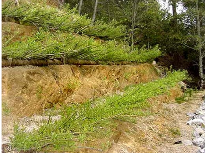
Figure 3.25 Brush Layering (Caltrans 2019b).
