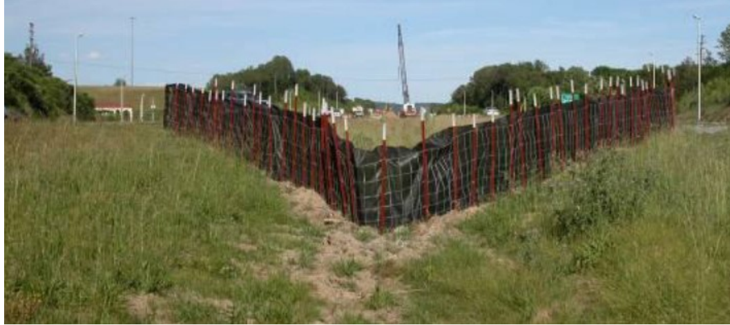
Figure 3.75 Reinforced Silt Fence (TDOT DM 2012b).
